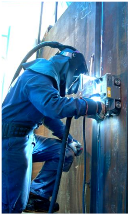
Vertical up butt welding using guide rail
